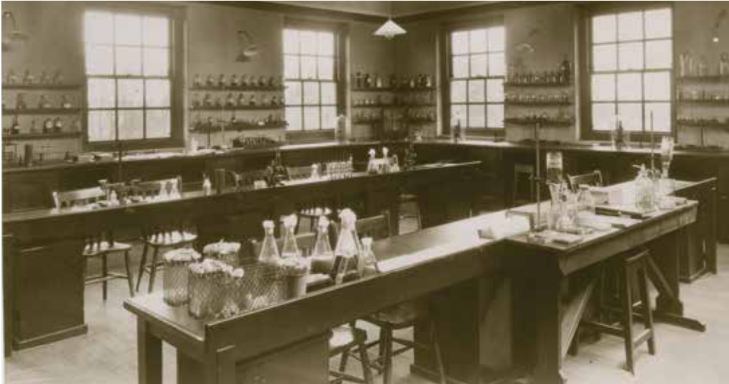
The Bacteriological Laboratory, in 1925; on the two benches are conical flasks, baskets for test tubes and stands holding filtration apparatus.
